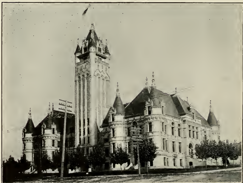
COURT HOUSE, SPOKANE, WASH.
